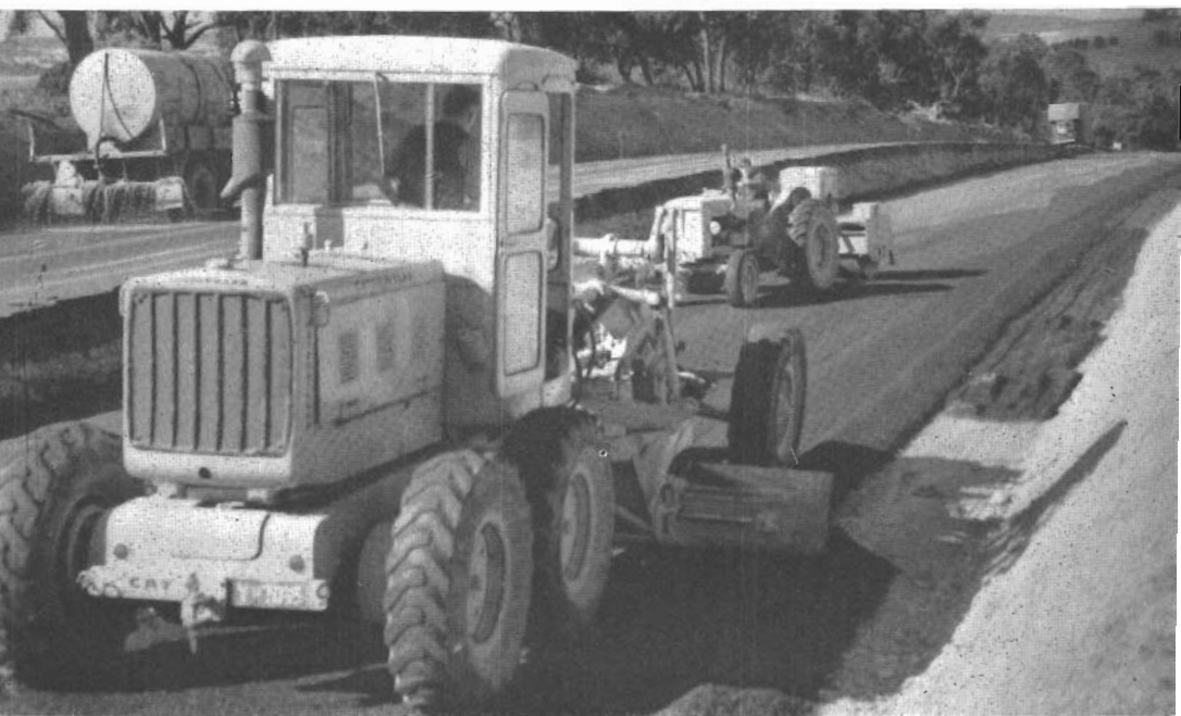
Reconstruction on the Hume Highway half-mile north of Wallan.
