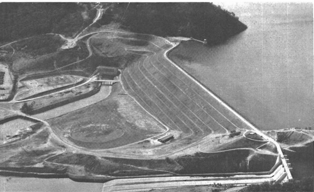
Aerial view of Eildon Reservoir and embankment at one end (foreground); spillway and power station at the other. The intake tower is just visible (centre) in the shadow of Mt. Sugarloaf. The Eildon boat harbor may be seen in the first inlet behind Mt. Sugarloaf
